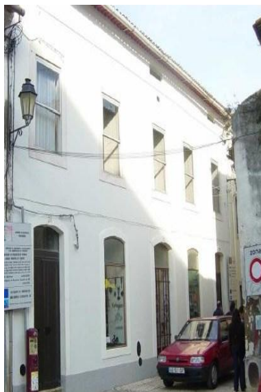
Figura 22: Rua da Nogueira, Coimbra – Portugal (Viva Coimbra, 2007)
