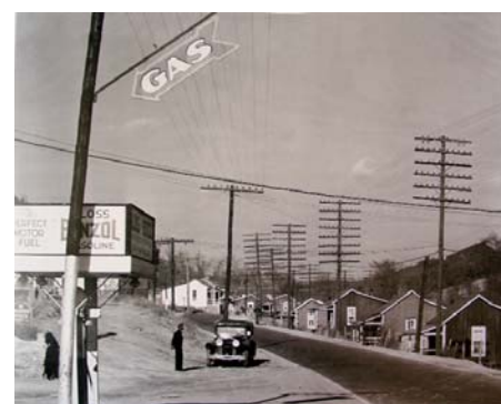
Walker Evans Roadside View, Alabama Coal Area Company Town 1936
