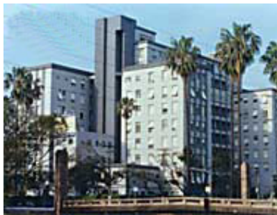
Figura 3.36: Vista Hospital Ernesto Dorneles
