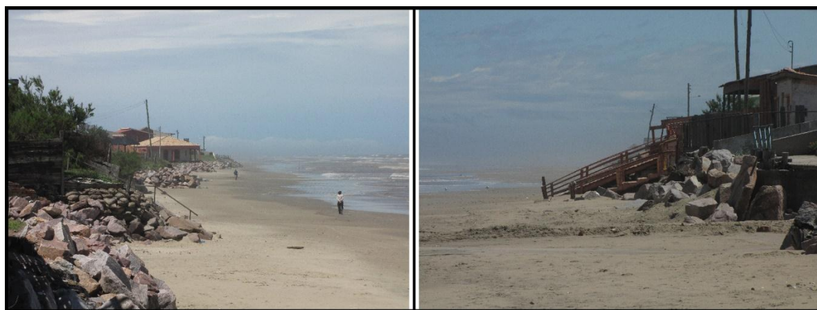
Figure 9: Damages done by coastal erosion in the Hermenegildo coastal town (Santa Vitória do Palmar) in the south coast of RS.
