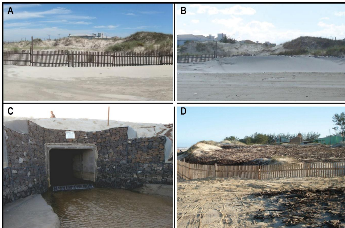
Figure 10: Foredunes recovery in the north coast of RS: A) beginning of the intervention to recover the foredune; B) sediments accumulated by the eolian transport; C) washout canalization to prevent dune erosion; D) dunes recovery above the canalization (A and B modified from Portz, 2012; C and D modified from Tabajara & Weschenfelder, 2011).
