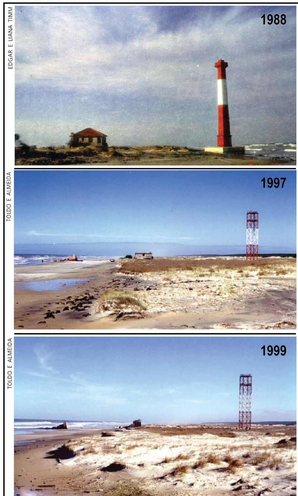
Figure 8: Coastal erosion on the Farol da Conceição location in the transgressive segment of the middle coast of RS. Photo from 1988 with the old lighthouse and the house behind; photo from 1997 with the old lighthouse destroyed; photo from 1999 with the house behind the old lighthouse destroyed (modified from Toldo Jr. et al. , 2006).
