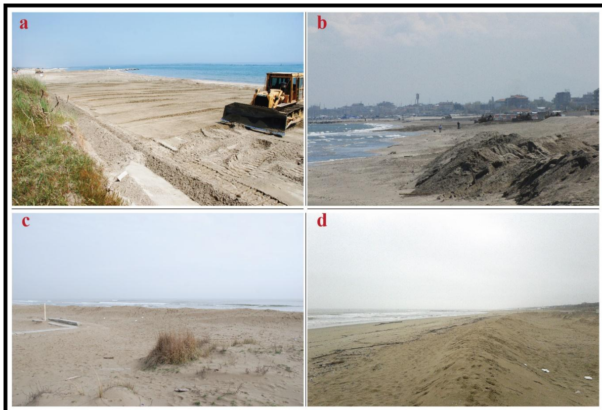
Figure 2: Bulldozer dunes; anthropogenic dunes built using a bulldozer on the Ravenna coast; a) bulldozer reworking the sand to prepare the beach for the summer season; b) bulldozer increasing the beach’s width for the summer season; c) behind a bulldozer dune in Marina di Ravenna during the winter season; d) above the bulldozer dune to protect the bagni .
