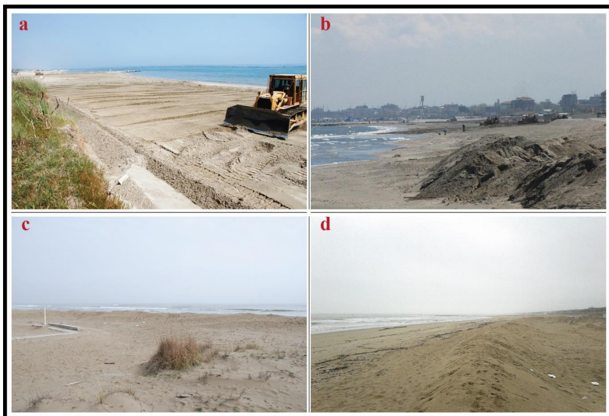
Figure 2: Bulldozer dunes; anthropogenic dunes built using a bulldozer on the Ravenna coast; a) bulldozer reworking the sand to prepare the beach for the summer season; b) bulldozer increasing the beach’s width for the summer season; c) behind a bulldozer dune in Marina di Ravenna during the winter season; d) above the bulldozer dune to protect the bagnini .
