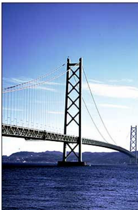
Figura 1.1: a ponte Akashi Kaikyo (fonte: Public Broadcasting Service ).
