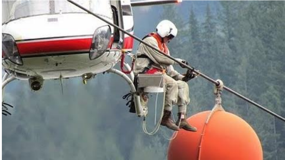
Figure 9 Power line inspection being doing by a man.
