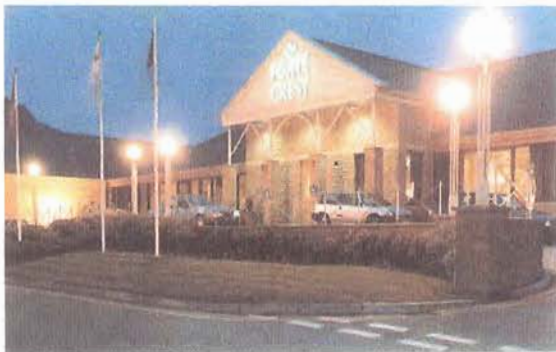
Figura 57 - Forte Crest Hotel, Brighouse, Reino Unido (BRECSU, dec.1994)
