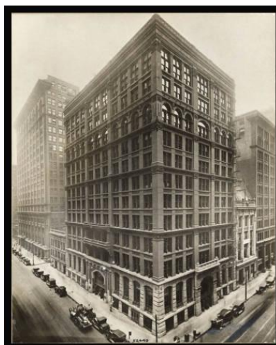
William Le Baron Jenney (1832–1907) Home Insurance Building, 1891 Chicago, Illinois, EUA The Art Institute of Chicago Ryerson & Burnham Archives
