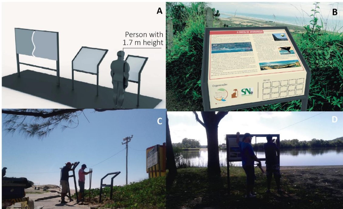
Figure 5: The creation process - panel installation of Araranguá Coast Geoecological Route Project. A) 3D model panels; B) Application of initial content, plotting the digital model layout; C) Panel structural fixing at Geoecological Interest Point; D) Adhesive bonding onto the panel support.
