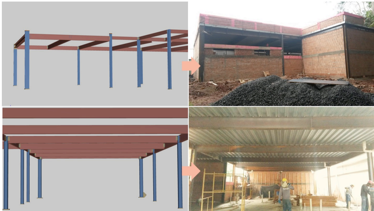
Figure 46: Instantaneous comparison of as-modelled and as-built
