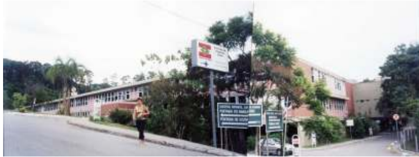
FIGURA 6.4 - Fachada principal do Hospital Infantil
