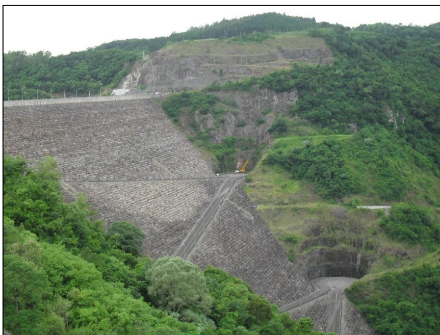
Figura 2-III- Campos Novos Hydroelectric Plant with concrete face. Source: Photograph taken by the author during the field trip on 11/26/2015.
