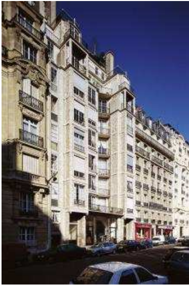
Figura 2. Perret, Ed. Rua Franklin, Paris, 1903
