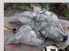
Fig. 142 Sun-O-House – Vista externa
