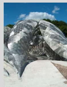
Fig. 138 Sun-O-House – Vista externa
