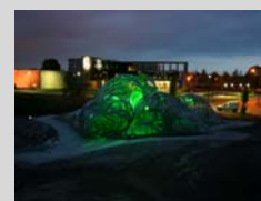
Fig. 134 Sun-O-House – Vista externa
