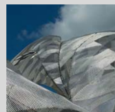
Fig. 130 Sun-O-House – Vista externa
