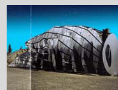
Fig. 146 Toilet Block Blowout – Vista externa
