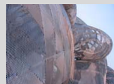
Fig. 133 Sun-O-House – Vista externa
