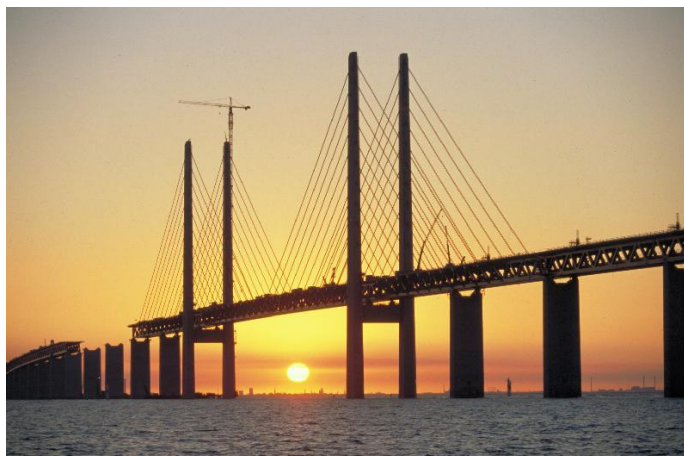
Figura 3.23 – Stonecutters Bridge (ARCILA, 2002).
