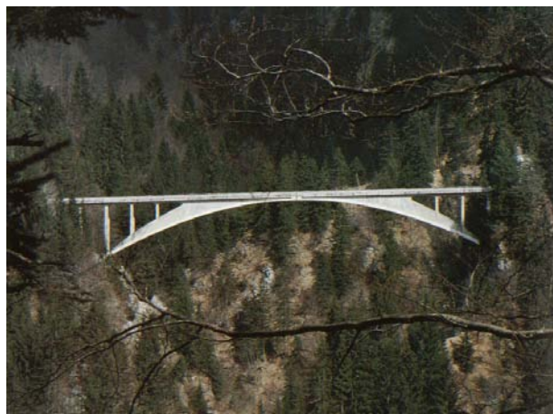
Figura 3.10 - Salginatobel Bridge (BILLINGTON, 1990).
