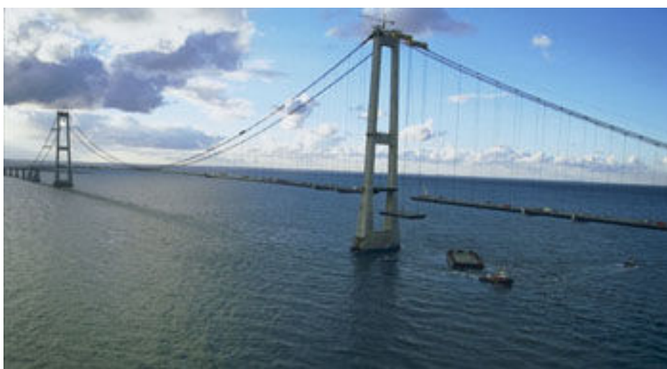
Fig. 1.18 – Ponte Great Belt East.
