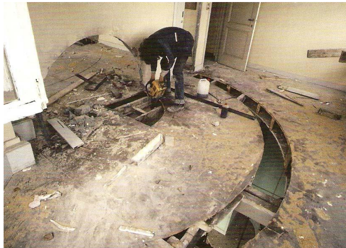
Figura 16: Gordon Matta-Clark realizando Office Baroque , 1977.
