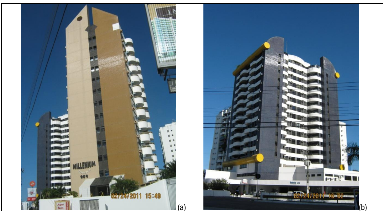
Figura 65. Millenium Residence (a) e Manhattan Residence (b)
