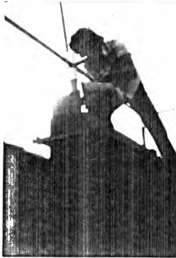
Fig. 3.58 - Self-Helper Filling a Form Using a Bucket
