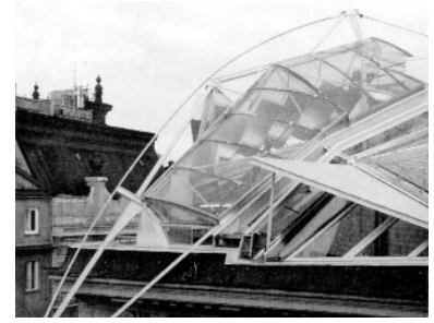
4.13.34 "Rooftop Lawyers' Office, Vienna, Coop Himmelblau, 1983-1988"
