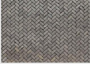
BLOCO INTERTRAVADO COM JUNTA SECA PARA FACILITAR A DRENAGEM NAS CORES BRANCO E CINZA INSERIDO EM TODO O CALÇADÃO DA ORLA
