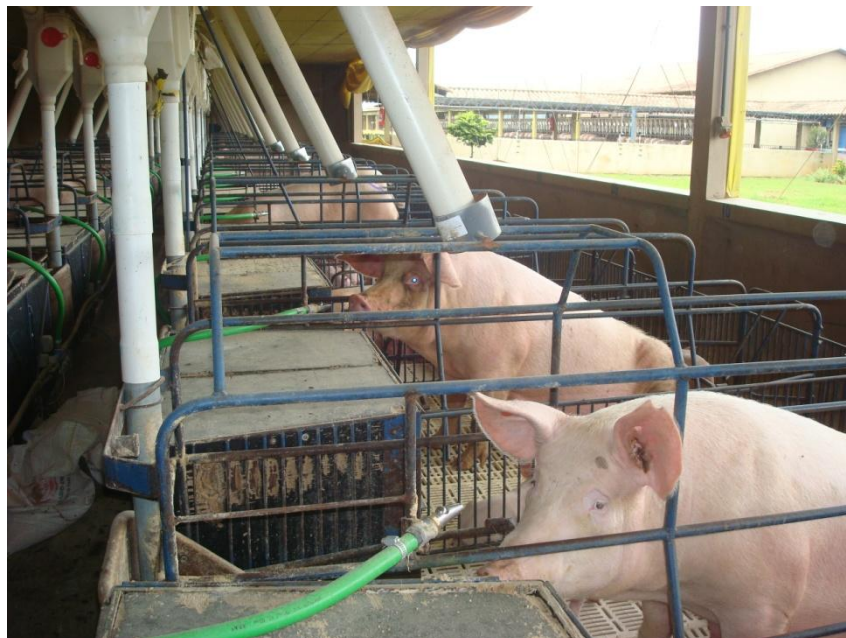
Figura 5B - Terminal ducts directing air cooled on the neck of sows
