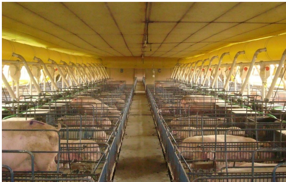
Figura 4 - Ducts independent distribution of cooled air the two lines of cells
