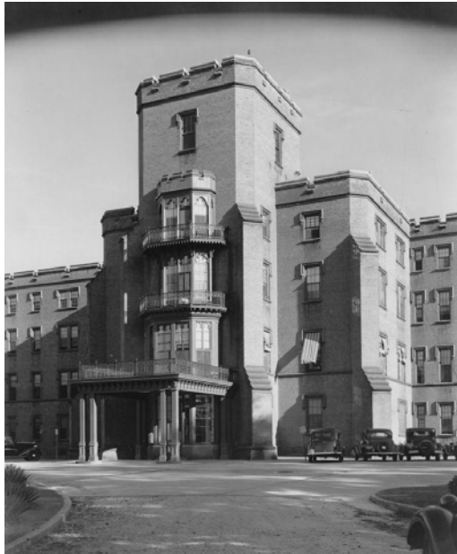
Figura 58. Hospital Saint Elizabeths. Edifício Central, 1938. Fonte: US, The Library of Congress. Photographs, written historical and descriptive data (...). Disponível em: http://lcweb2.loc.gov/pnp/habshaer/dc/dc1000/dc1099/data/dc1099data.pdf
