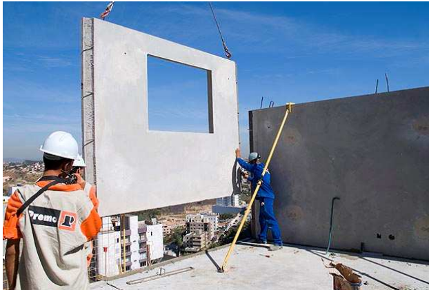
Figura 22 – Painel de concreto
